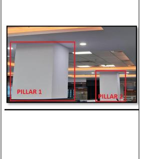
Size of Pillar: 3.5ft x 8.5ft (WxH) Each face of Pillar for LED installation: 3.6ft x 4.9ft (WxH)
